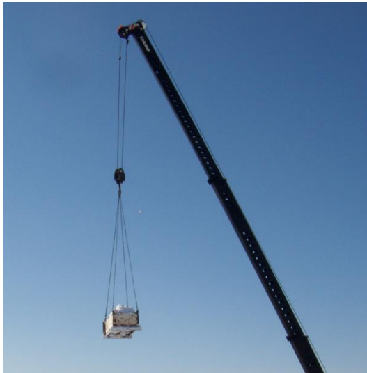
Crane and hopper removing snow (Photo source: Zurich)
