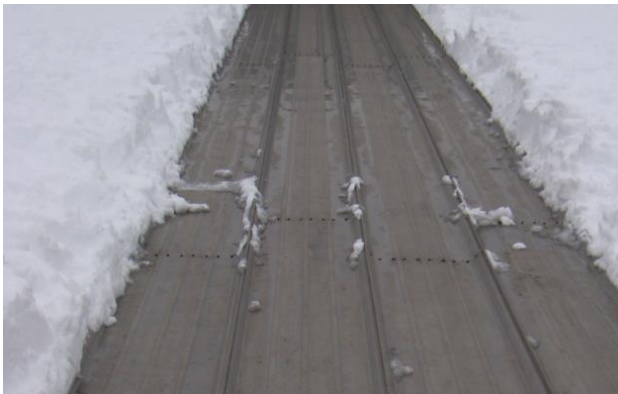
Snow removed from center of bay (Photo source: Zurich)
